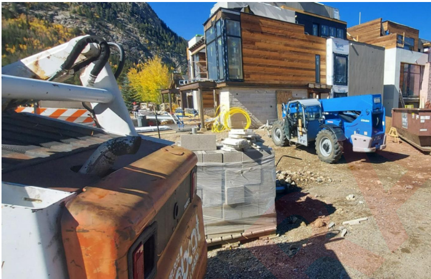
Multi-family home construction project in Frisco, CO. VertSites 2023.
